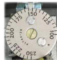
Set-point dial protected within a NEMA 3R enclosure
